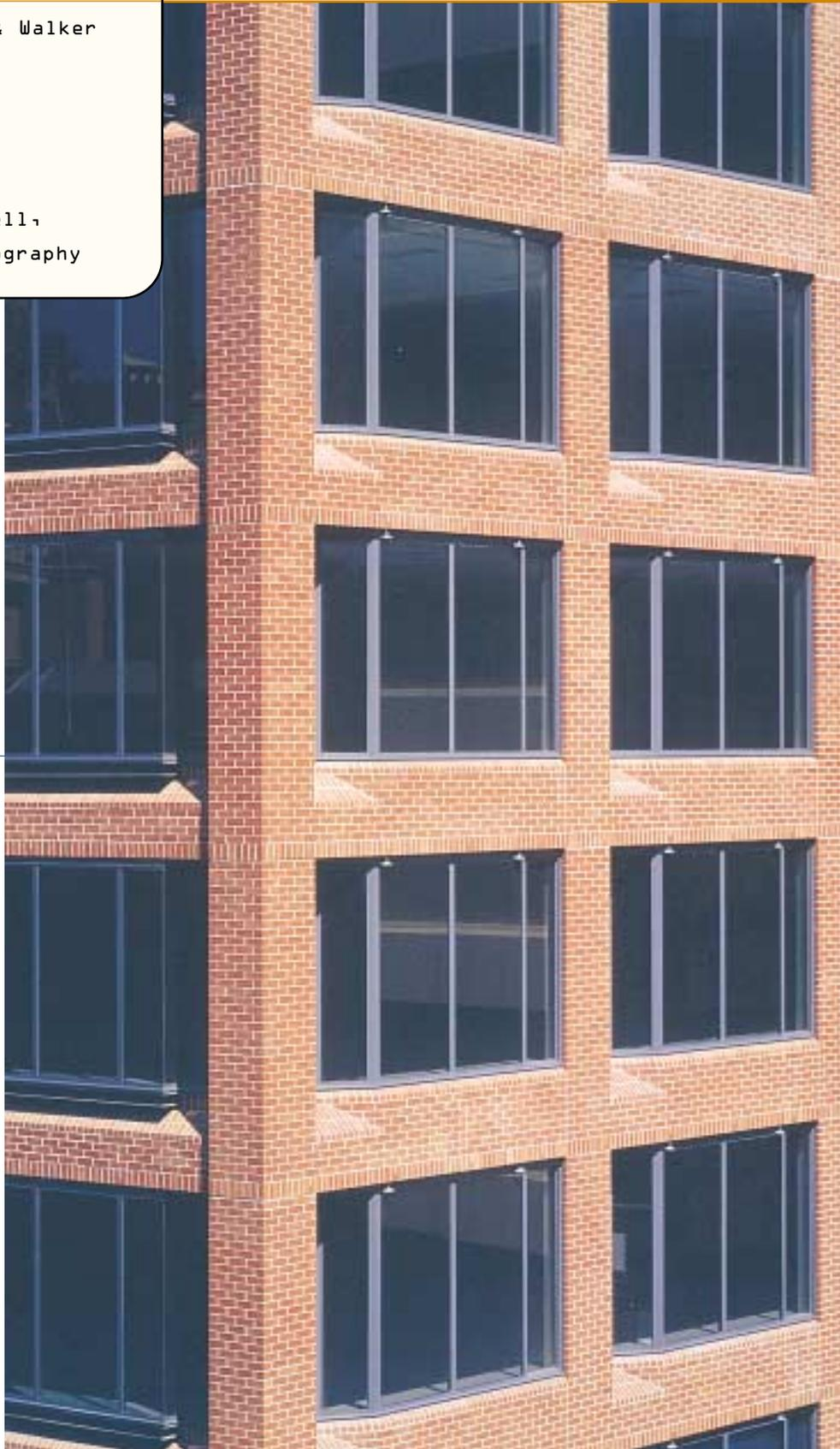
(Above) The brickwork detailing of deep reveals and sloping sills creates the framework for the bay window glazing. A test panel provided invaluable data to the designers and builder.
