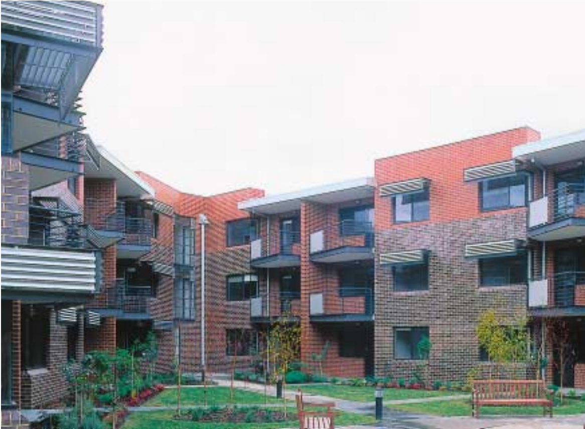
The inner units look out over the landscaped, north-facing courtyard. The structure is predominantly loadbearing with clay bricks in the outer leaf.
