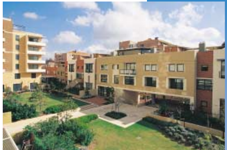
(Above) Stage 3 utilises a mix of face and rendered brick to impart a sense of individuality and diversity.
