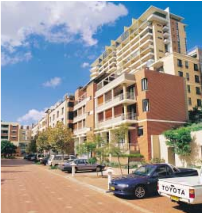
The brick paved internal street is "one of the most successful aspects of the whole project" according to the project director. The pavers are laid in a 45 degree herringbone pattern on a concrete base with sand-filled joints.
