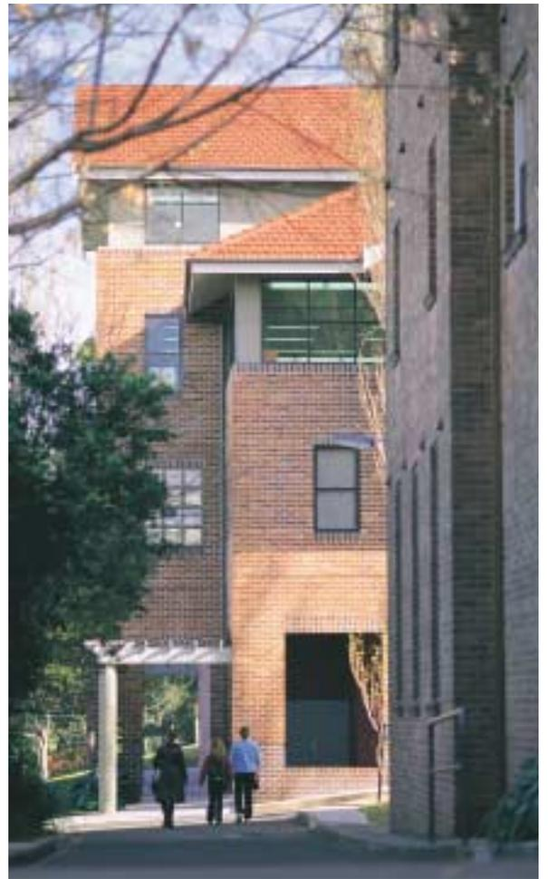
*(Top) The eastern elevation clearly shows the new building abutting the old. The building is firmly based in red/blue brickwork, the colour being repeated in arches, heads and sills.*
