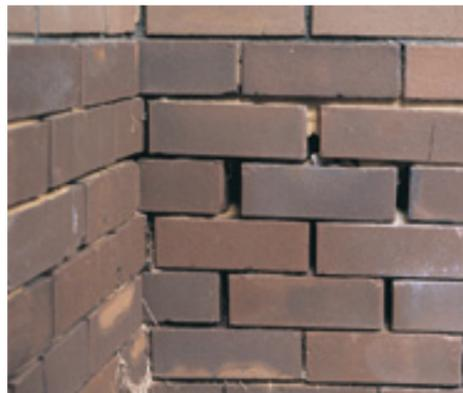
*Salt attack may cause a weak mortar to crumble or a non-durable masonry unit to spall, as these extreme examples show.*
