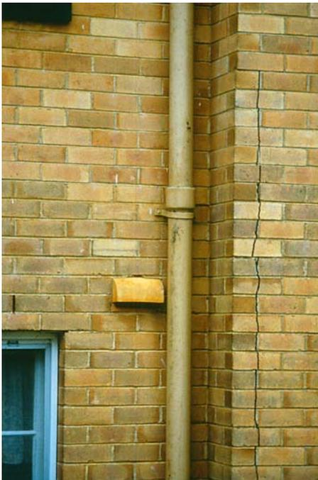
**Figure 5. Cracking at re-entrant corner**
