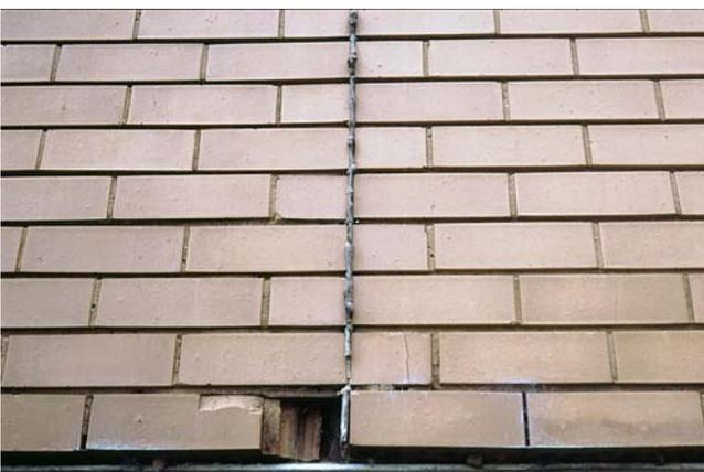
**Figure 6. Extrusion of expansion gap filling material due to inadequate gap width**
